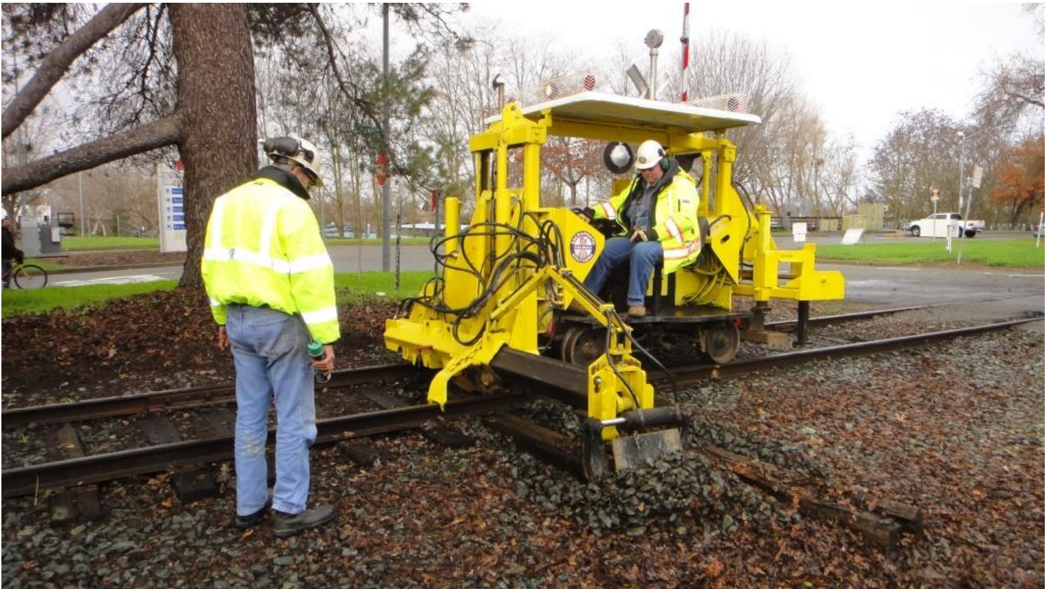
Alan marks ties for Chris C. in the Jackson 125 tie-exchanger to pull out...
