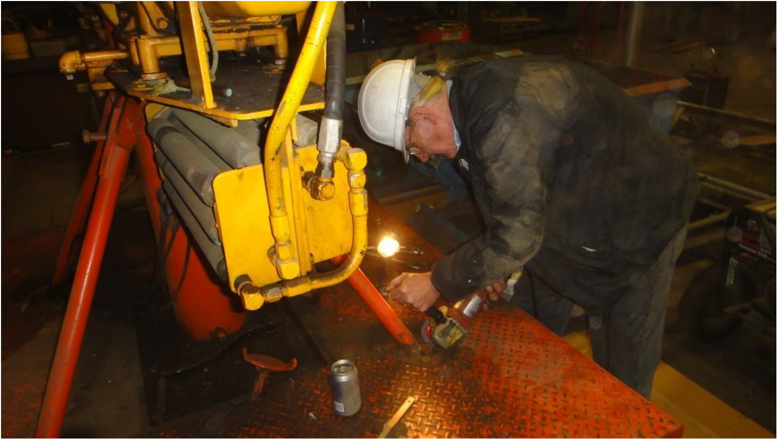
Fred takes on removing the derrick crane's support brackets
