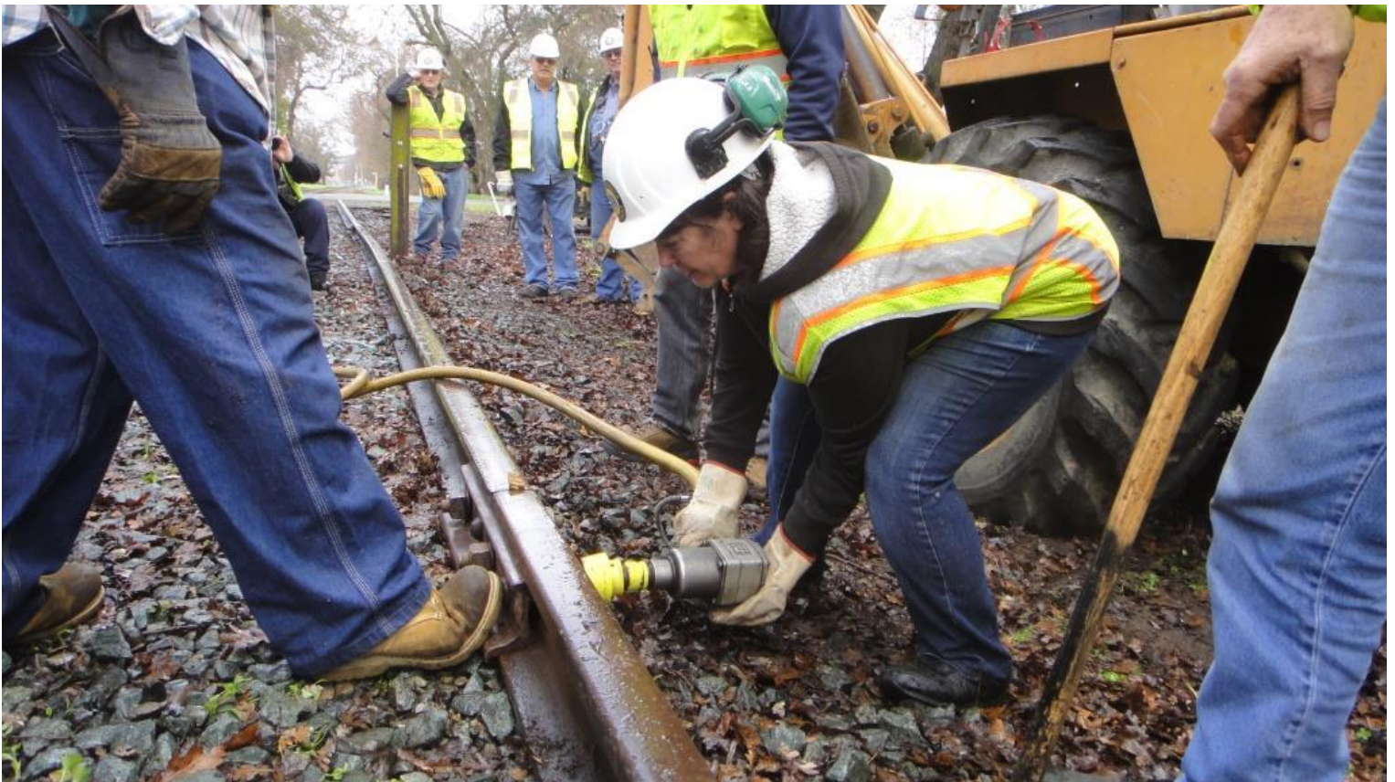
Pam with the pneumatic impact wrench tightens bolts extra tight
