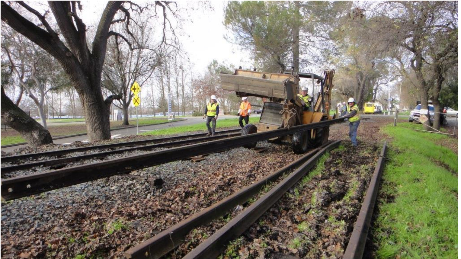
Steve N. guides the next rail into position. That's nearly 1,500 pounds of rail Harry is moving with the back-hoe
