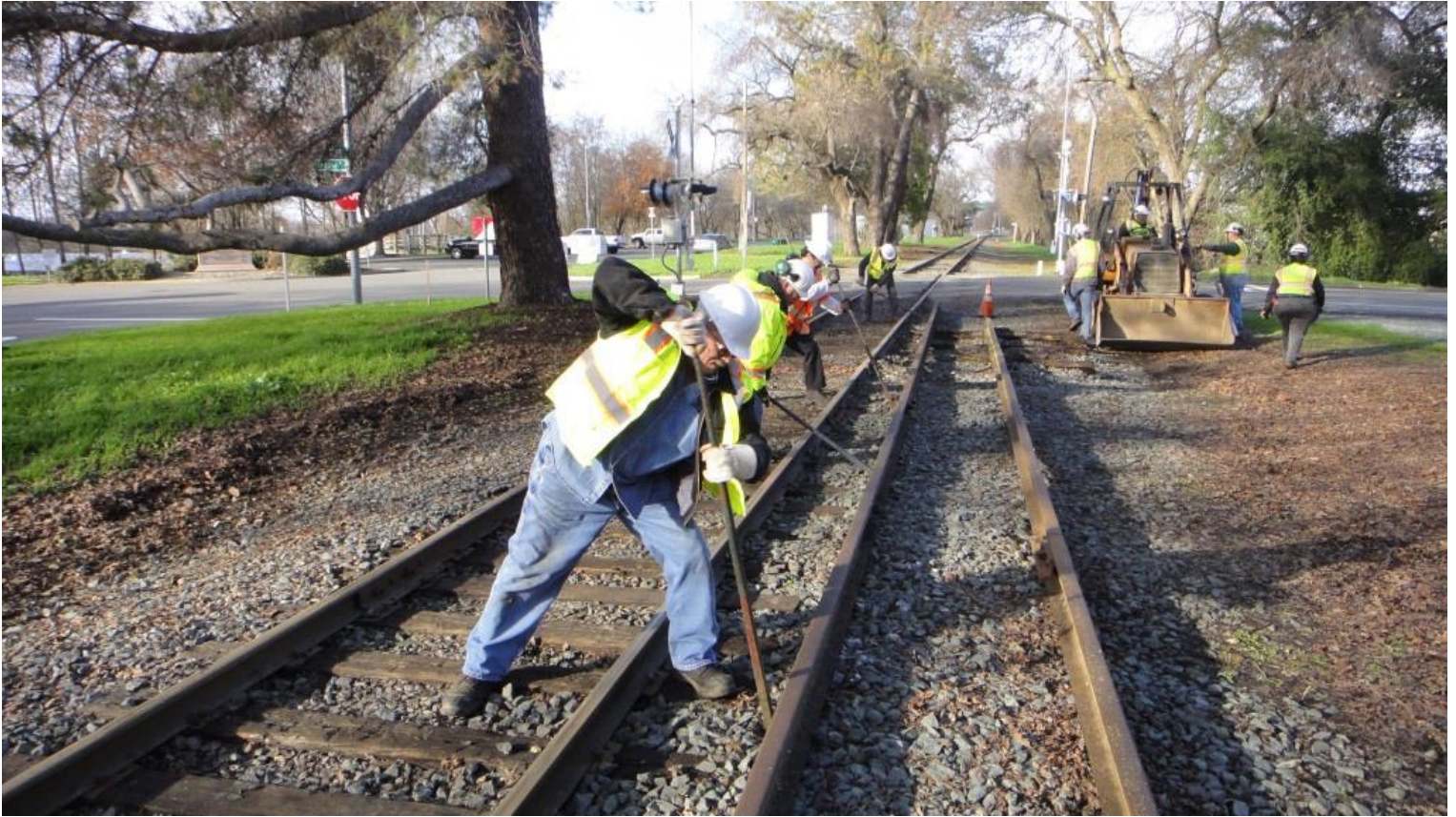
Gandy Dancin': The Team uses lining bars to move the replacement rail away from the track
