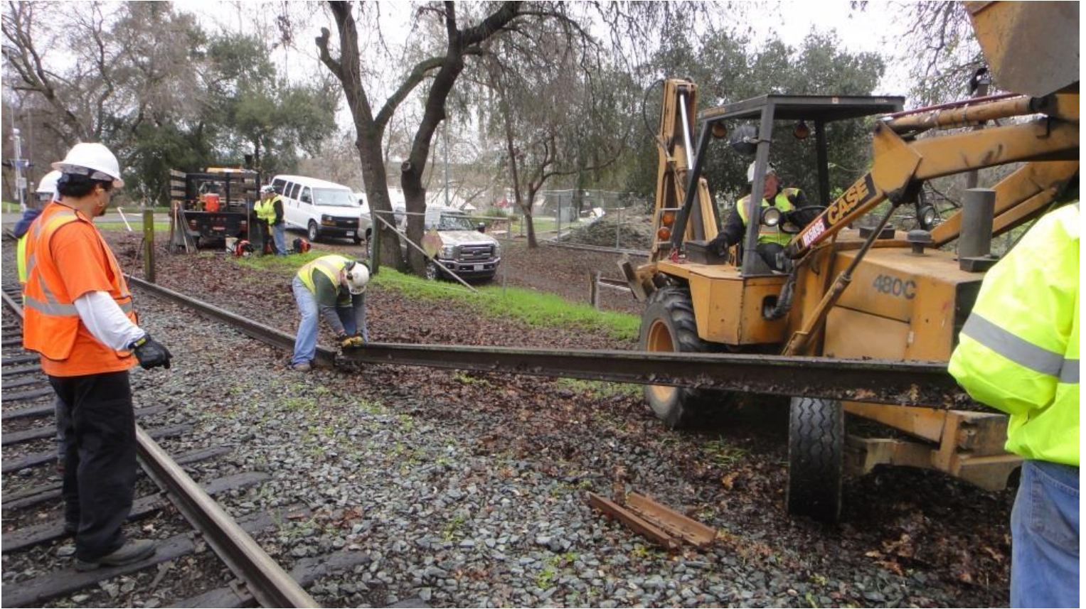
Mike F. lines-up the rail-ends of the new rails that Harry in the back-hoe positions
