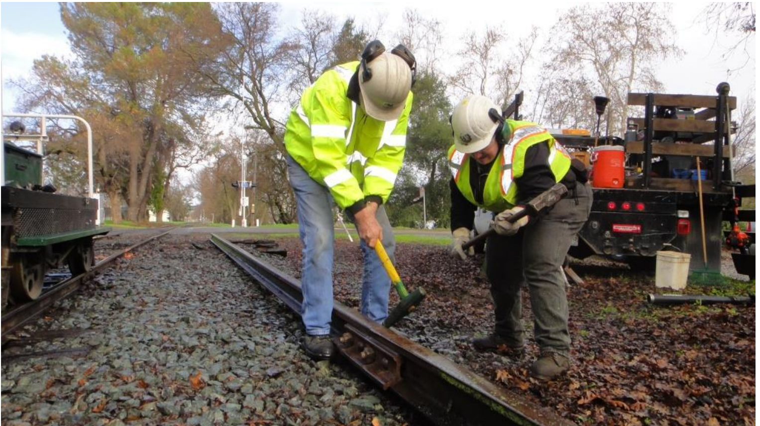
Alan and Heather chisel-off bond wire welds
