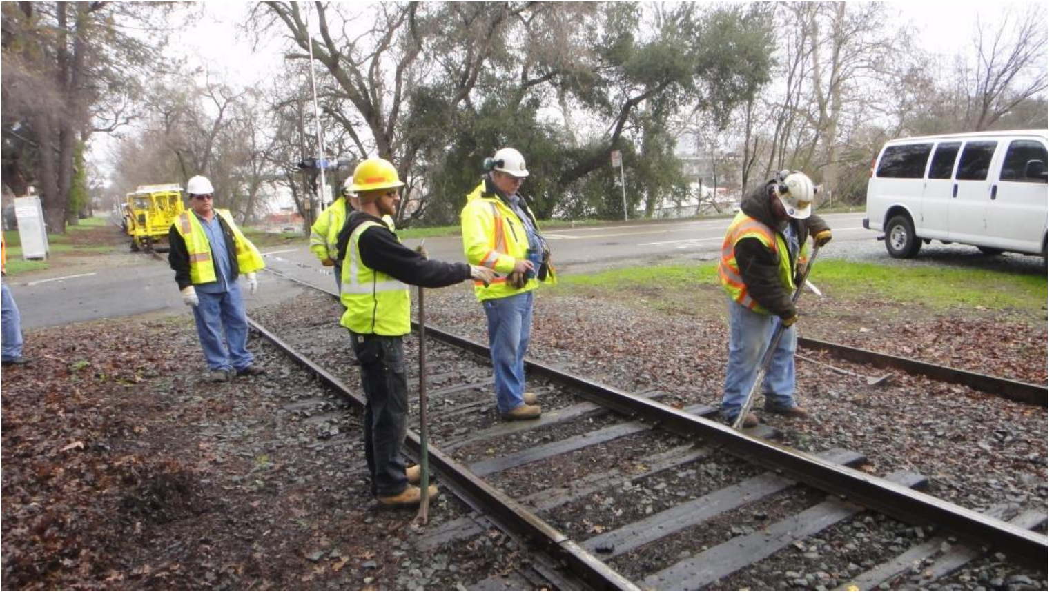
Chris M., and Mike F. start pulling spikes
