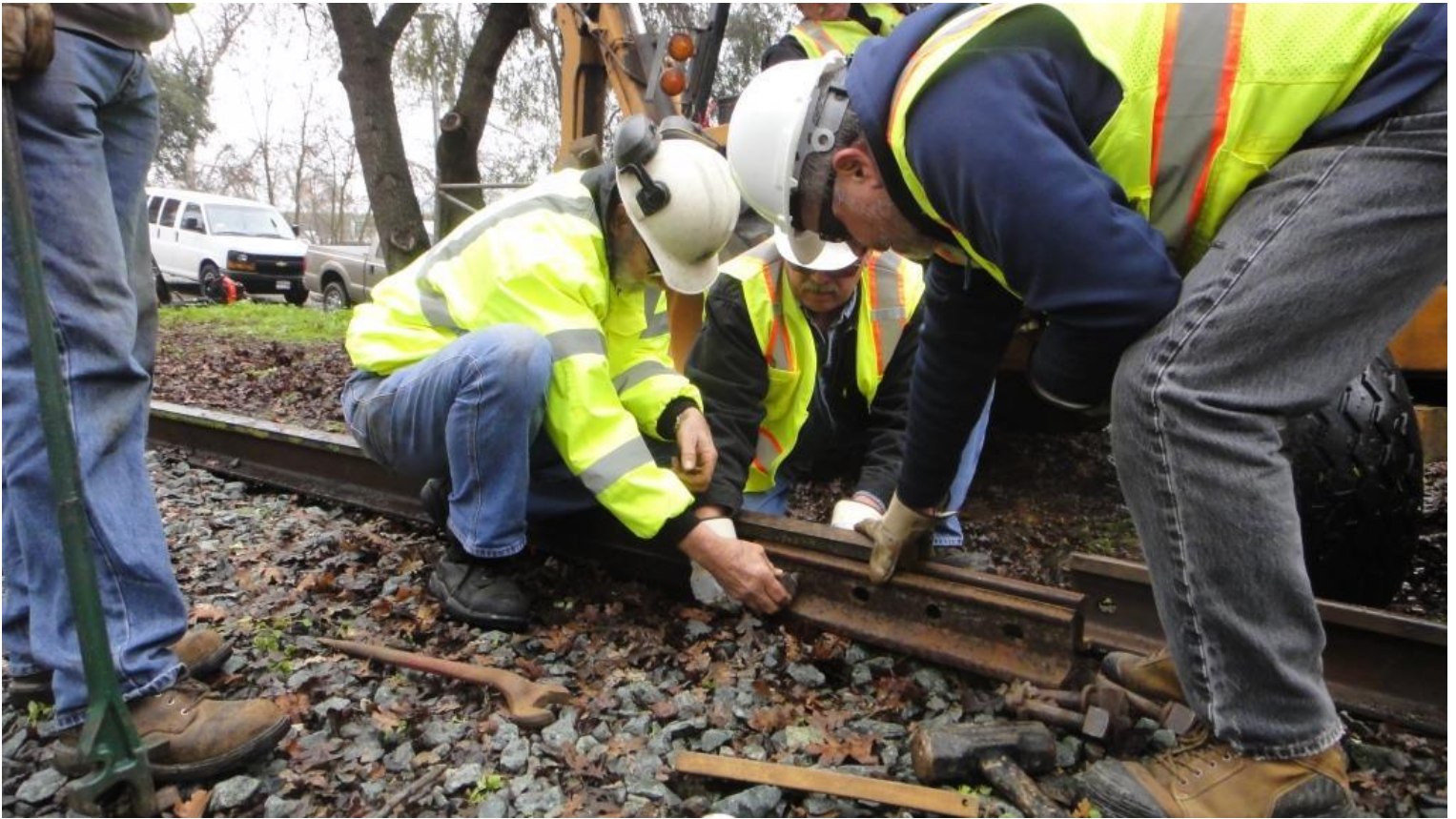
Alan, Scott, and Steve W. position the joint-bars at the next rail
