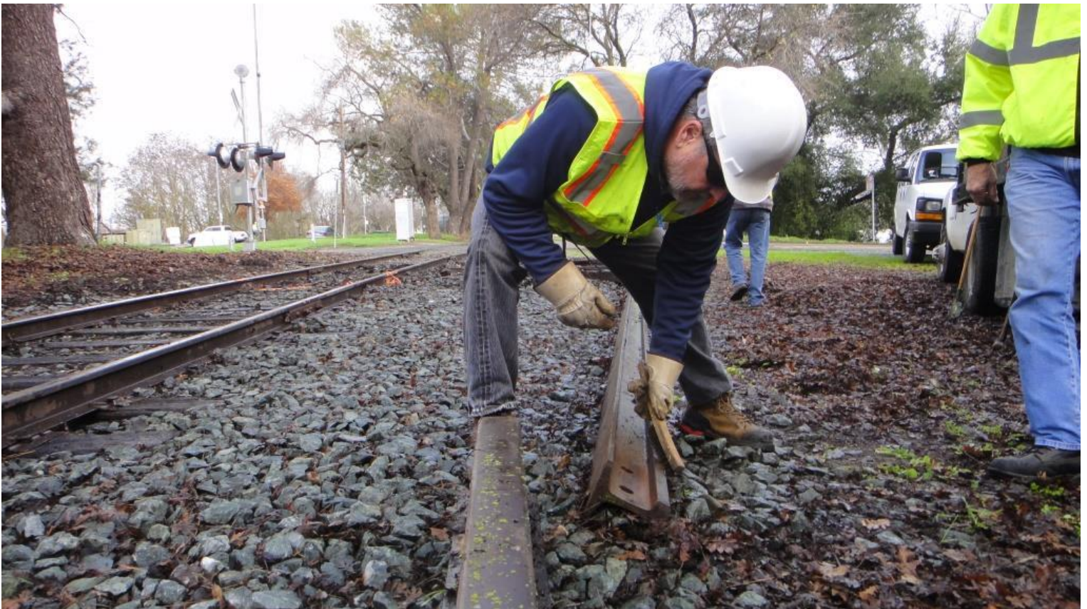
Steve W. cleans of the end of a rail...
