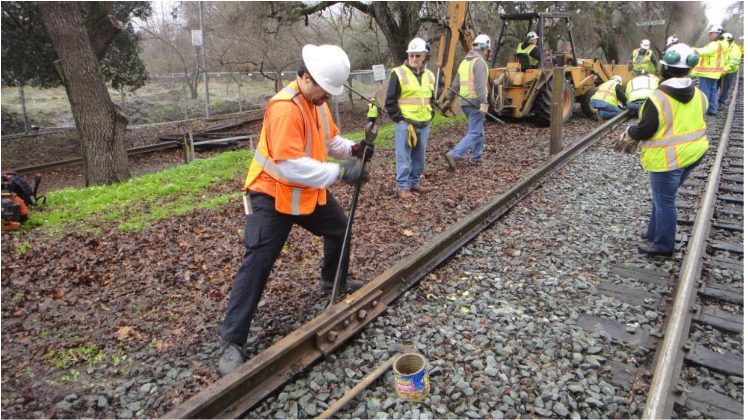
Jose first tightens-up the bolts with the track wrench...
