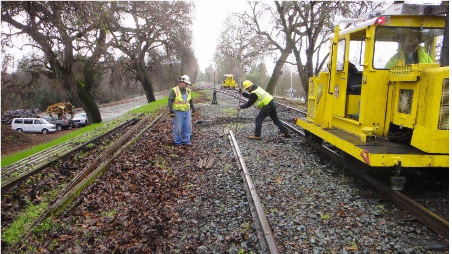
Chris M. pivots the rail with a lining bar to align it with the joining rail
