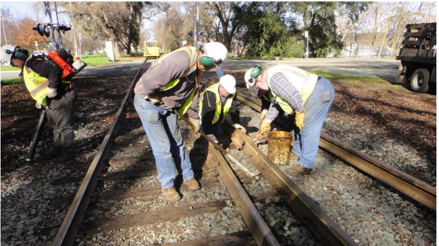
Steve, Scott, and Frank apply grease behind joint-bars before they are bolted up. Heather continues the organic debris dispersal
