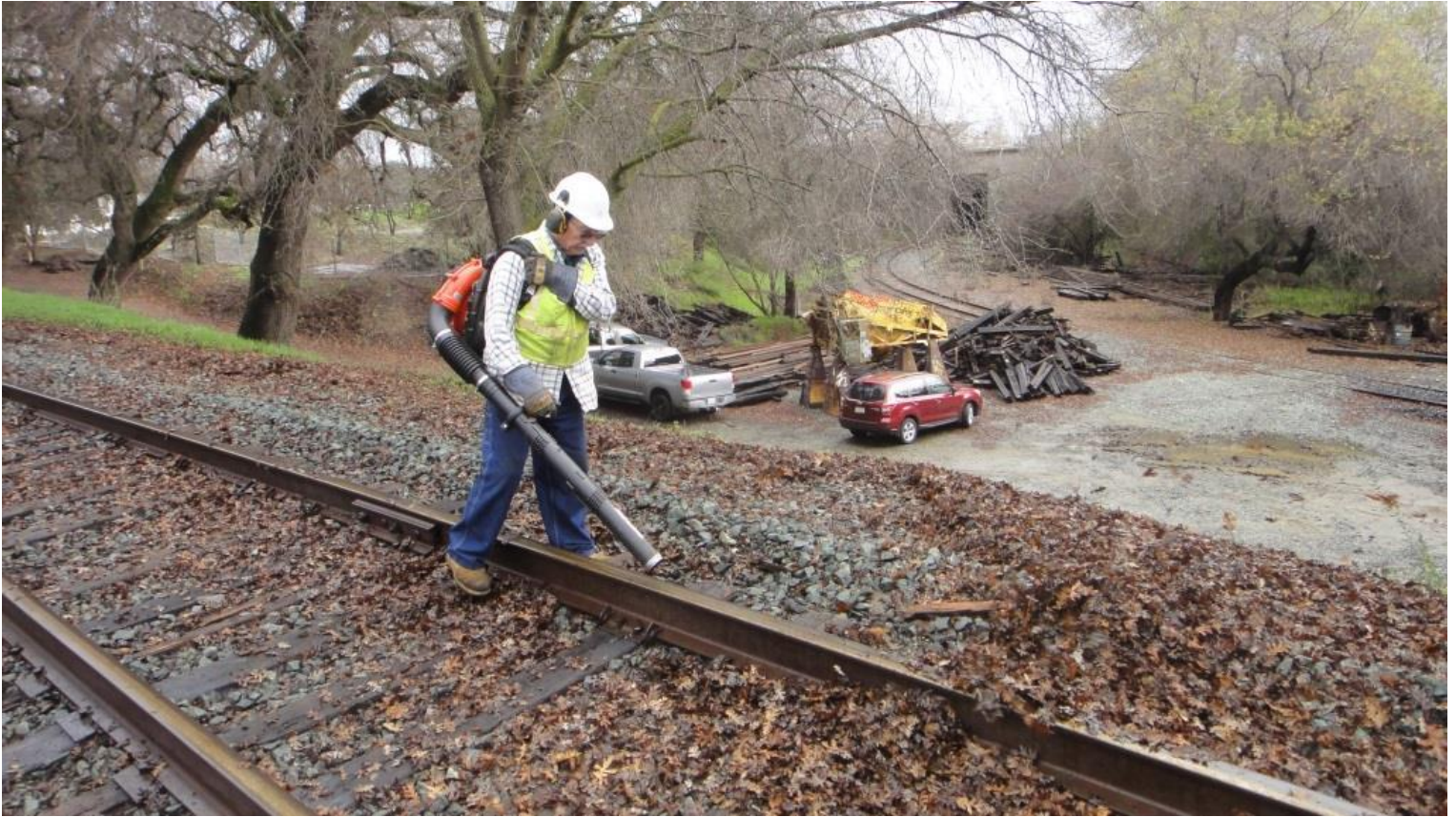
Clem forcibly removes organic debris occupying the track
