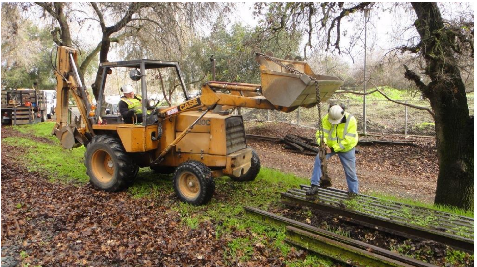
Alan attaches the rail-tongs to a stick of 110-lb. rail which Harry in the back-hoe will drag into position
