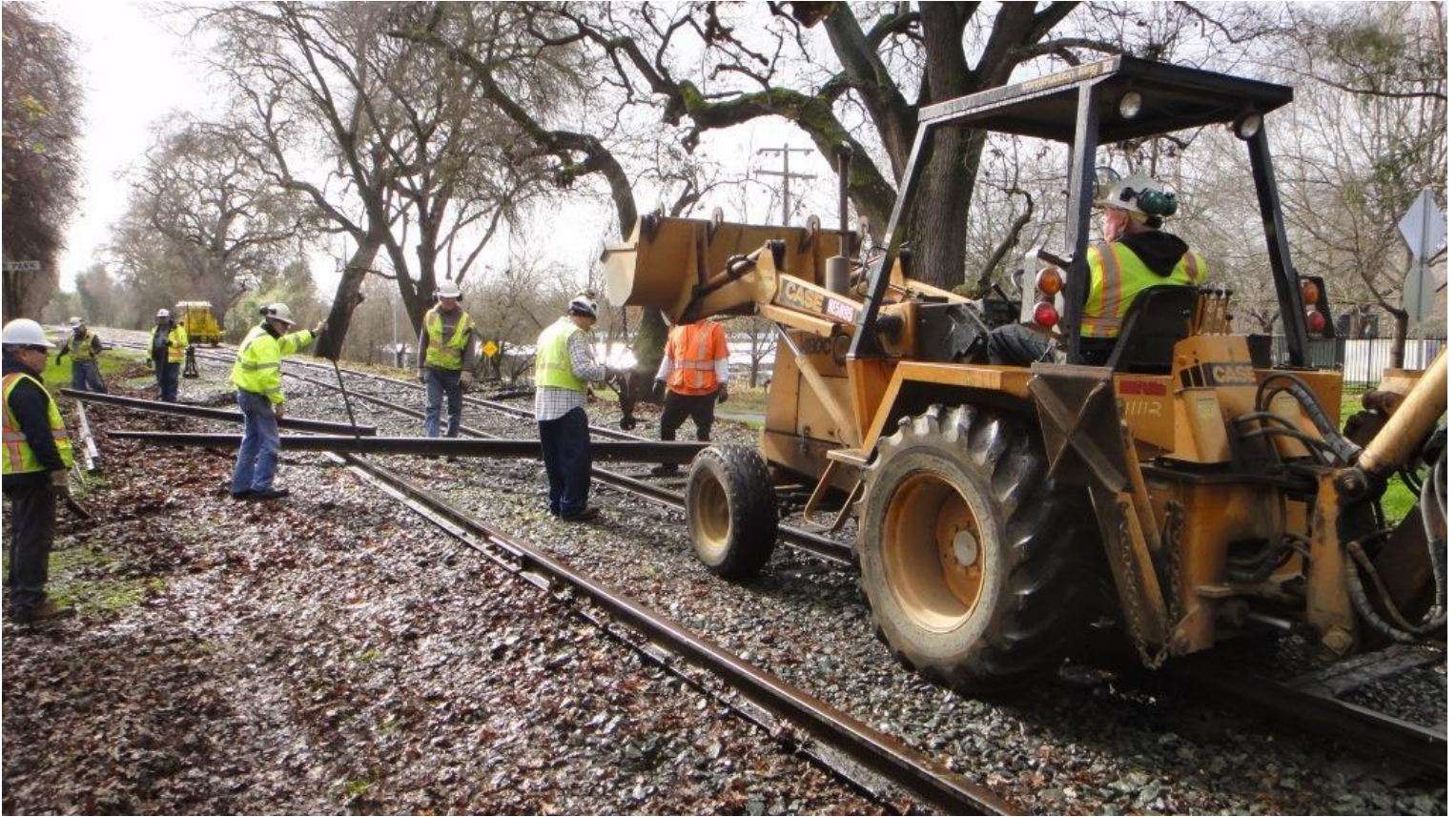
Harry pulls the first rail for the west side into position
