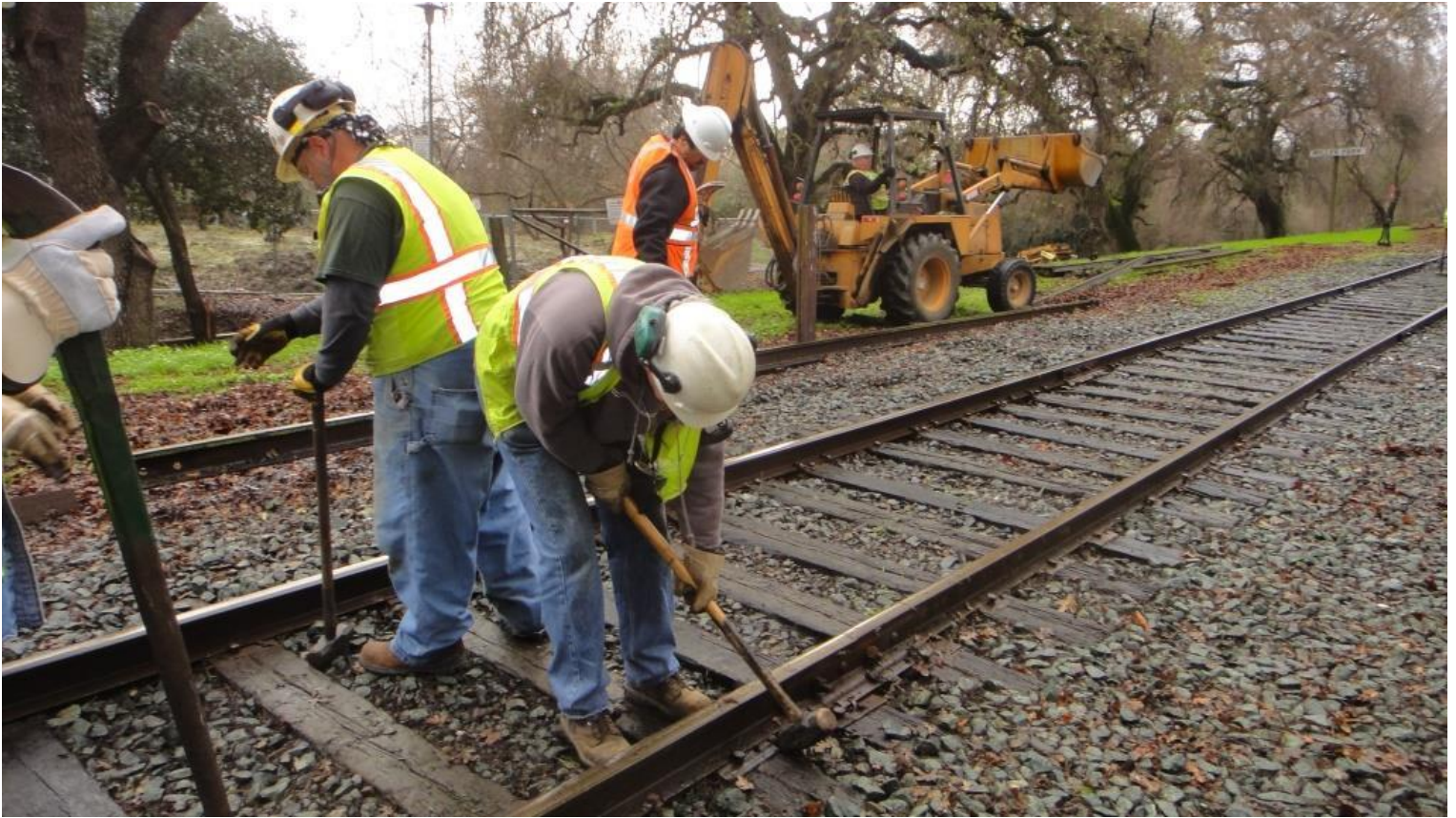
Mike F. and Steve N. remove rail-anchors
