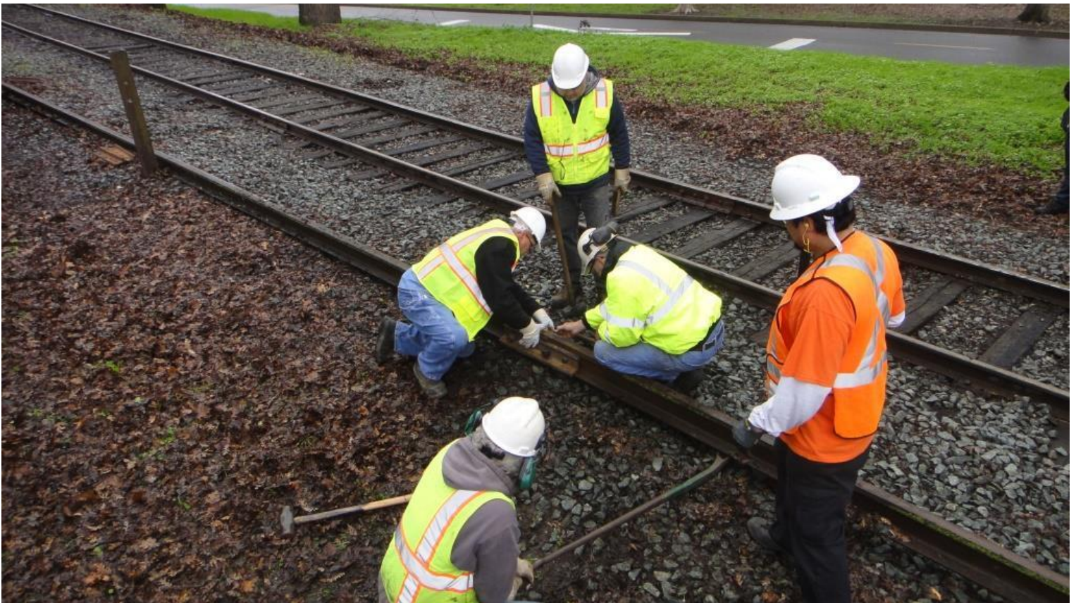
Steve N. nips up the track while Scott and Alan apply joint-bars
