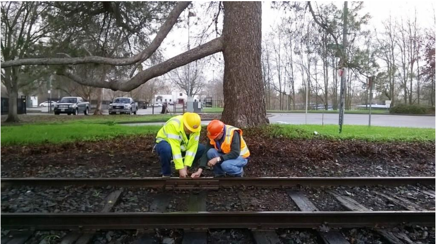
Marc Pryor and Dale Parker remove bond-wires in the south approach at Front Street
