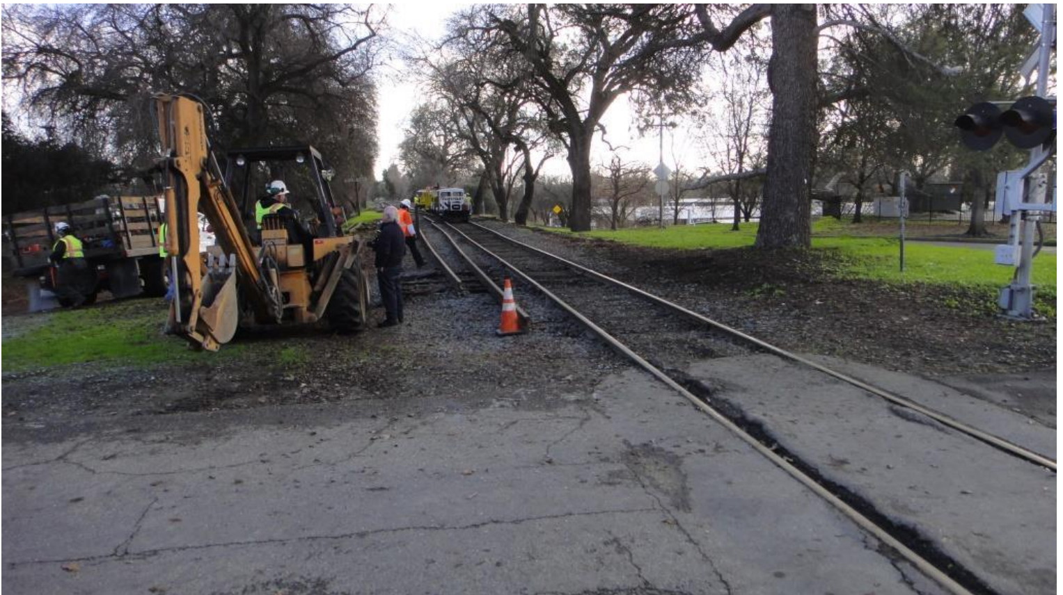
The tidied-up work-site as we pack up to head back to the Shops
